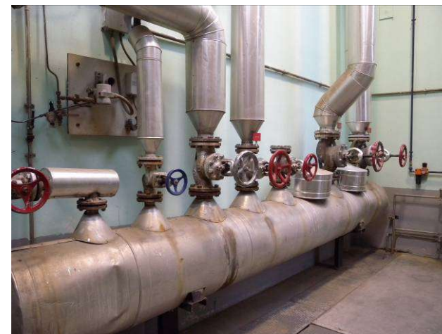
Insulated steam pipe
